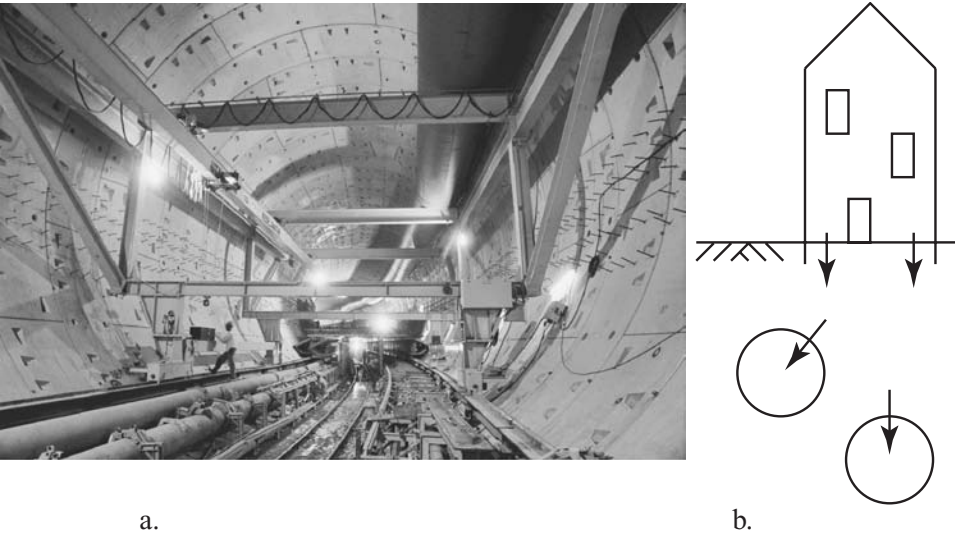
Figure 1.4. (a) Combined flood relief and road tunnel under construction (Kuala Lumpur, Malaysia) (©Mott MacDonald); (b) tunnelling beneath existing foundations.
