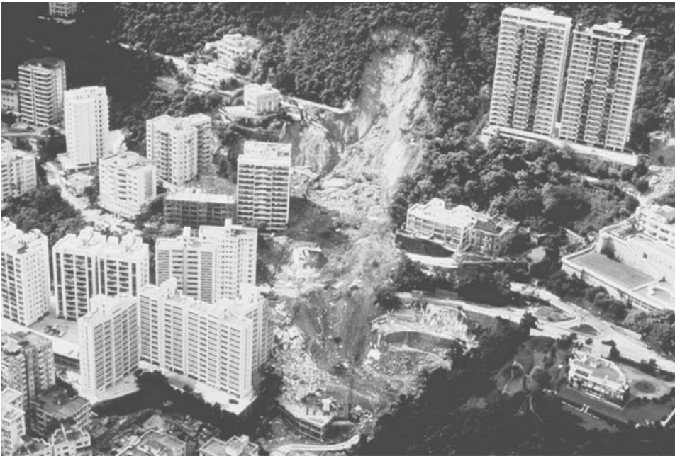
Figure 5.2. Slope failure in Hong Kong triggered by heavy rainfall (Po Shan Road, 18 June 1972) ( http://hkss.cedd.gov.hk/hkss/eng/photo_gallery/Landslide/index_1.htm ).
