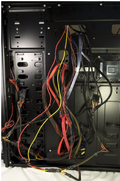
Figure 5-75. The cable management area, before dressing
