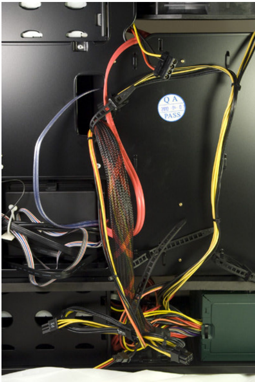
Figure 4-64. The hidden rats' nest of cables
