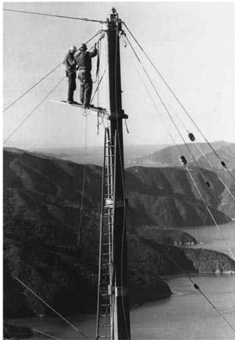
Construction of the tower to support the power cable across the Tory Channel in the Marlborough Sounds, New Zealand (Source: Neil Rennie)
