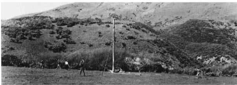
A Wellington Municipal Electricity Department pole gang erect a hardwood pole, New Zealand, 1935 (Source: Neil Rennie)
