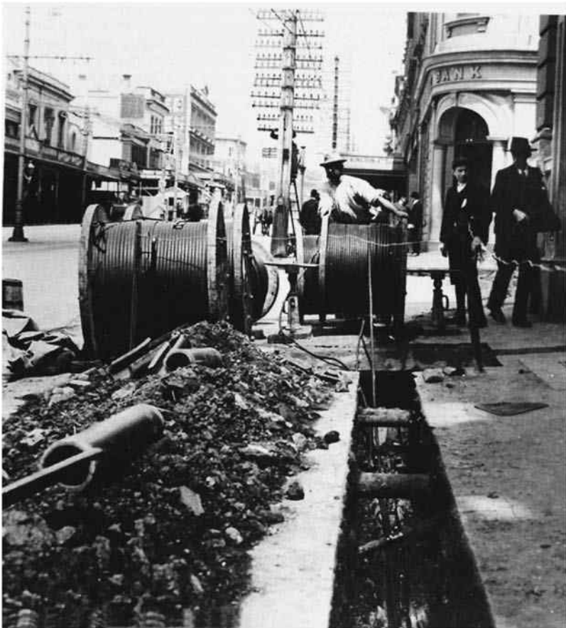
Laying cables for the Auckland City Council's power distribution system, ca 1908 (Source: Neil Rennie)
