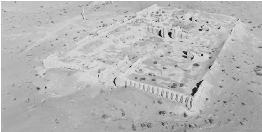
Figure 12.2 Kite photograph of one of the best-preserved architectural sites in the survey area (KRS20): the caravanserai known locally as Akcha Kala (white castle) (photograph by Alexis Pantos).
