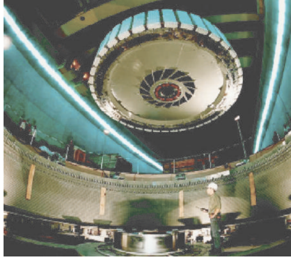
Figure 1. Hydro-generator during installation of the rotor.
