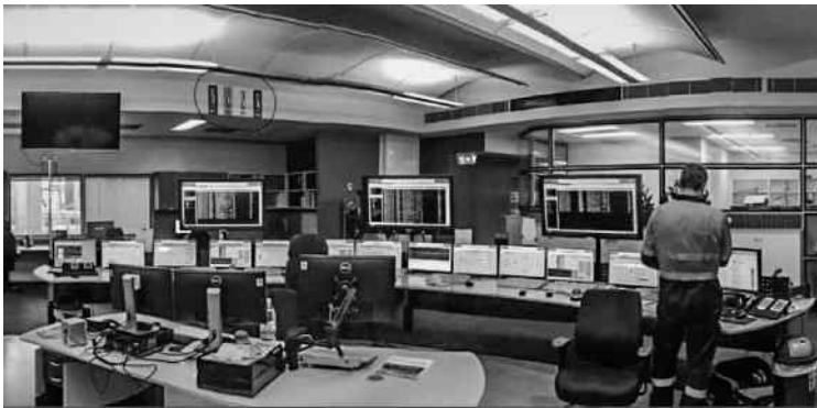
Figure 12.3 New control room for the four-unit gas-fired plant. Control consoles for four other units of an adjacent station were also located in the same room. Note the 'Yarway' drum level indicators (circled). © AGL Energy Ltd. Used with permission
