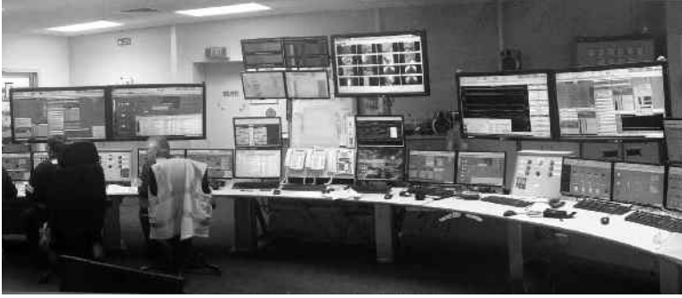
Figure 12.5 Replacement HMI for both units and common (station) plant, located in a different area of the same control room. © Millmerran Operating Company. Used with permission
