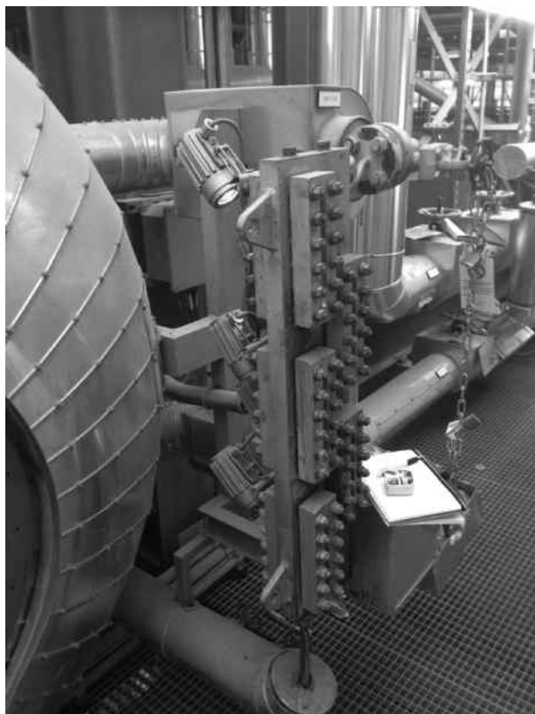
Figure 6.21 Drum-level gauge. © TC Fluid Control, a part of WIKA Instruments, reproduced with permission
