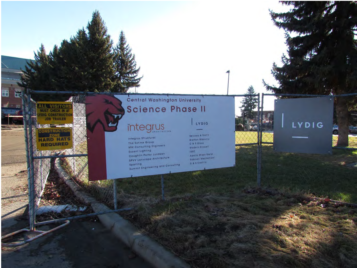
Figure 10-4: Example of visitor signage at the project entrance that instructs all visitors to report to the project office (Picture Courtesy of Lydig Construction)
