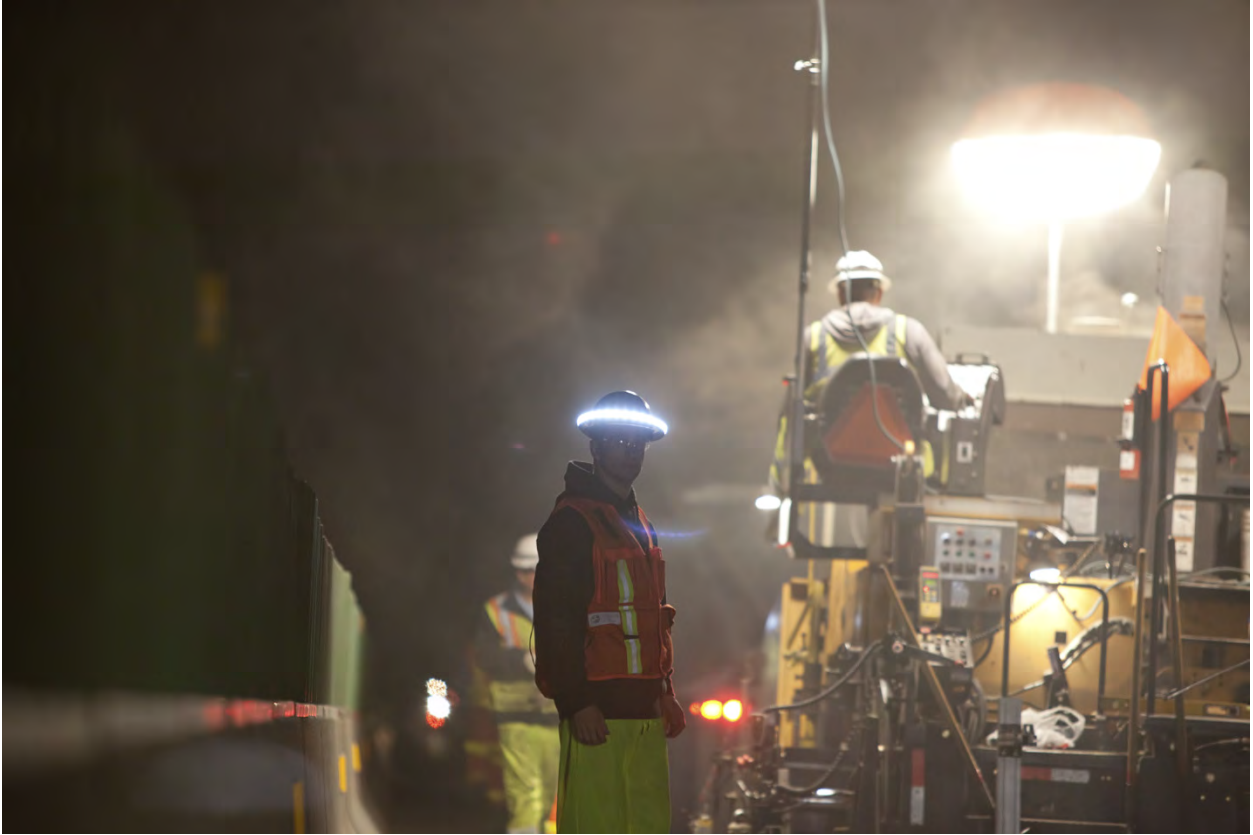
Figure 8-5: Halo Light – An example of Personal Active Safety Systems (PASS) (Photo courtesy of ILLUMAGEAR)
