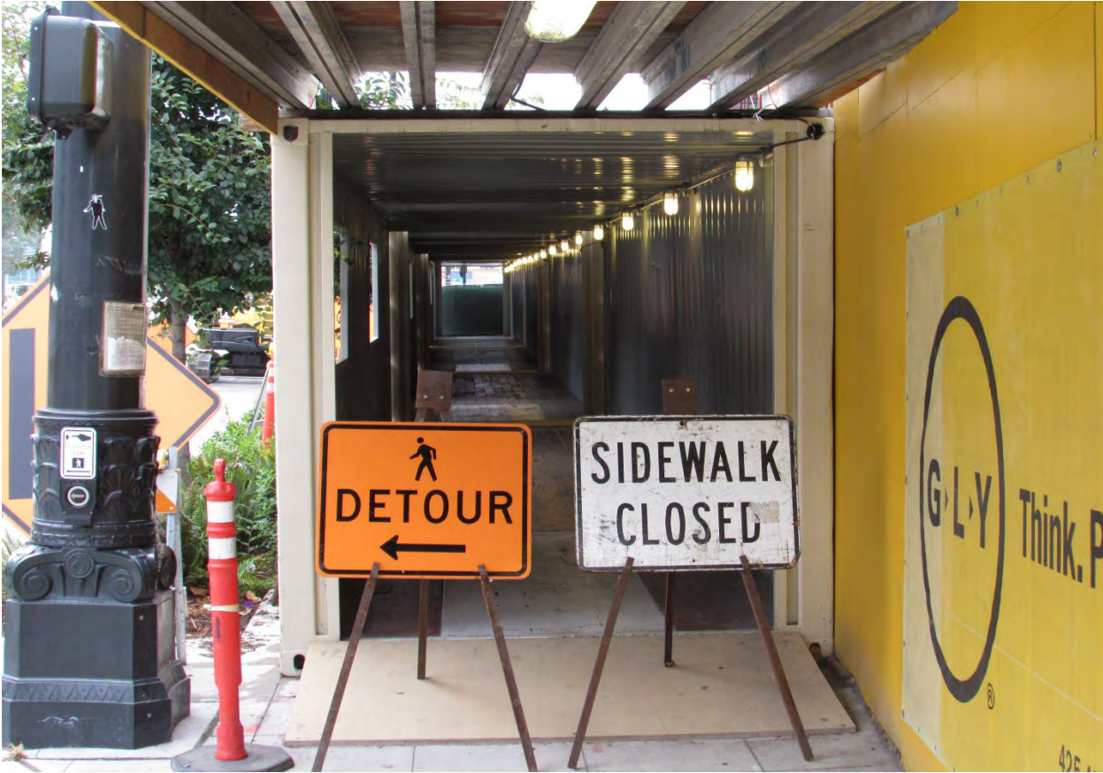
Figure 10-8: Example of Pedestrian Pathway and Falling Object Protection around construction sites (Picture Courtesy of GLY Construction)
