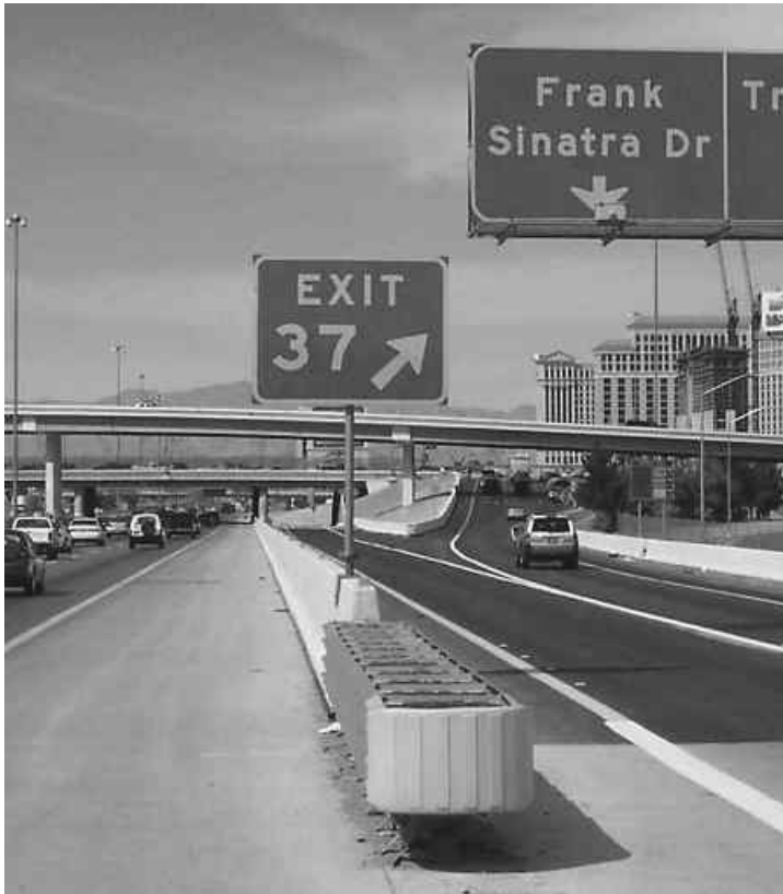
Figure 14-4. Example of an energy-absorbing guardrail (the QuadGuard system). Telescoping sections collapse when impacted and crushable, foam-filled cartridges absorb energy. (Photo provided by Quixote Corporation, Chicago, IL.)
