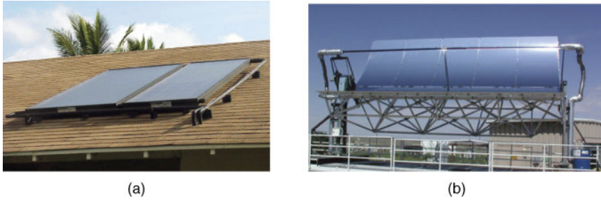
Figure 7.1 Examples of flat-plate and parabolic-trough solar collectors: (a) flat-plate (NREL 09188); (b) parabolic trough (NREL 14087).
