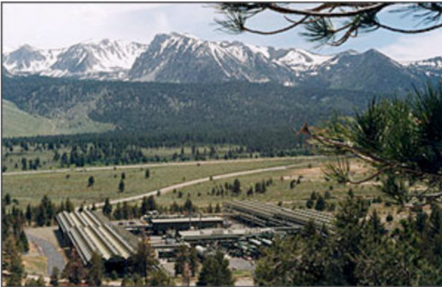
Figure 13.18 Mammoth Pacific I, a binary geothermal power plant. Source: EERE.
