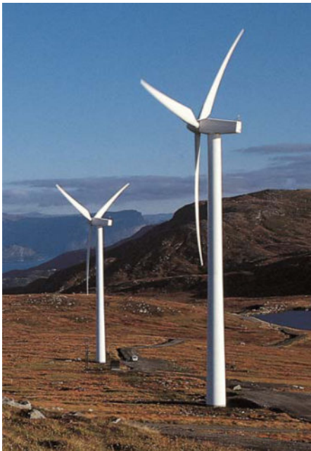
Figure 4.23 Vestas V52 850 kW wind turbine. Source: http://images.nrel.gov/viewphoto.php?imageId=6311986 .
