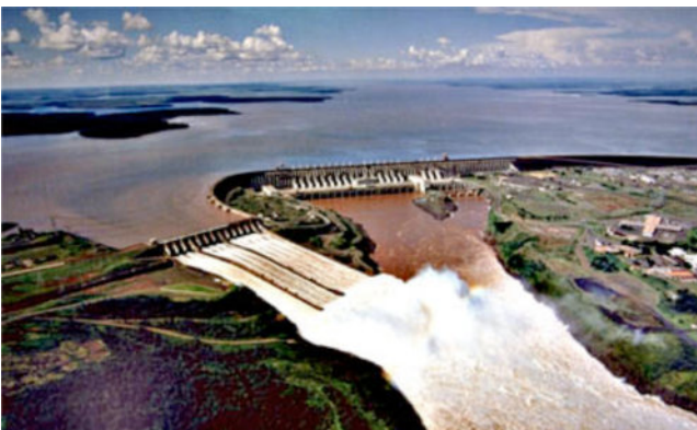
Figure 3.4 Aerial view of the Itaipú hydroelectric power plant.
