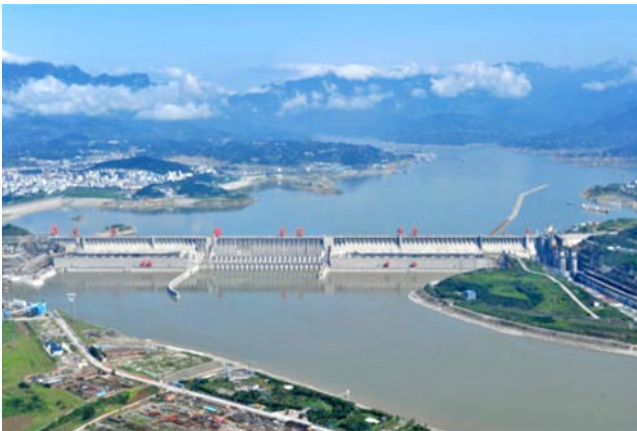
Figure 3.5 Three Gorges Dam. Source: Power Engineering International (November 17, 2014).
