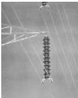
FIGURE 5.7 Creepage Extenders Installed in a Transmission Line. Courtesy of Tyco Electronics.
