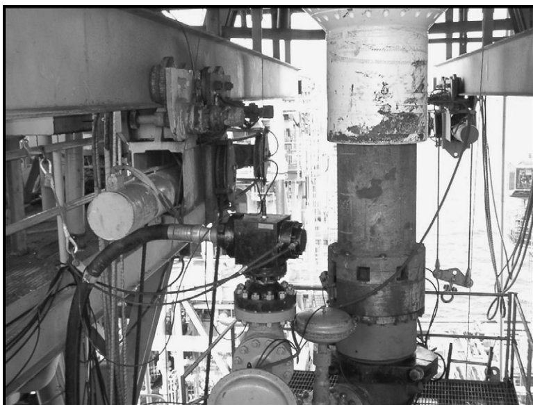
Figure 3.5 The HOLD 2500 rotating control head being installed in a wellhead on a deepwater offshore platform in the Gulf of Mexico. (Courtesy of Smith International, Inc.)
