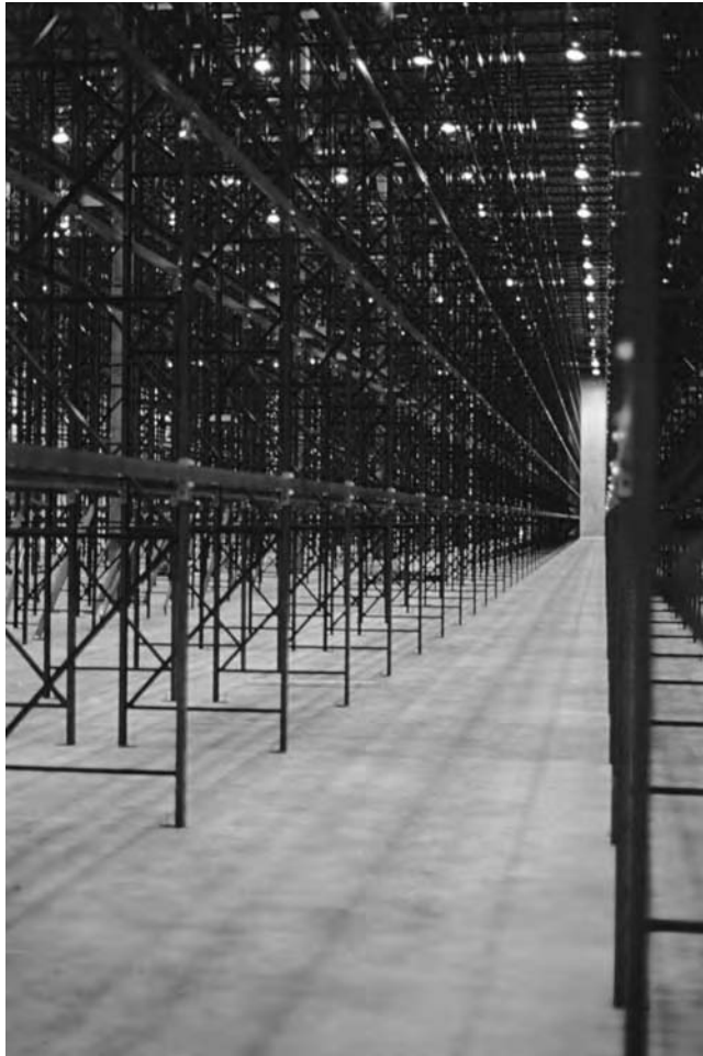
Figure 5.4 Pallet racks impose concentrated loads
