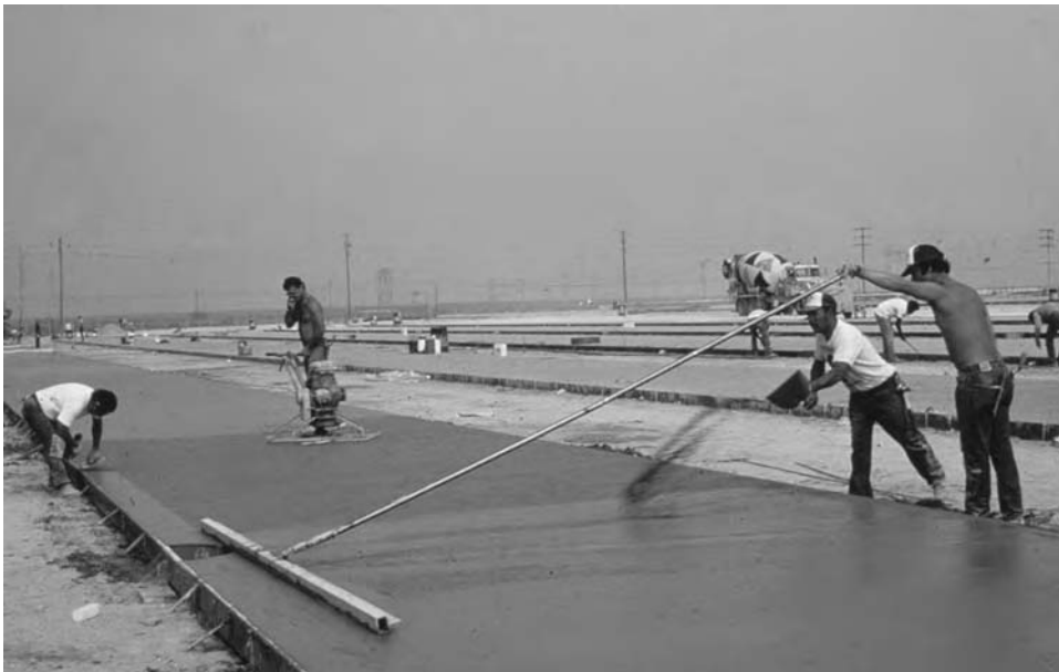
Figure 17.2 Highway straightedge
