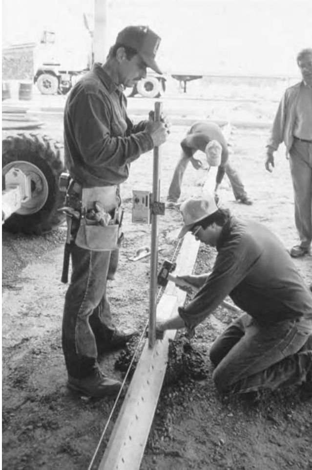
Figure 11.9 Using a laser to set precast concrete screed rails
