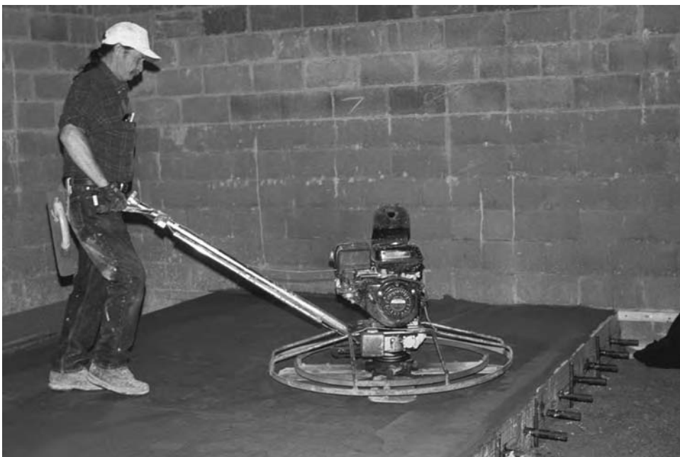
Figure 17.6 Walk-behind power trowel machine
