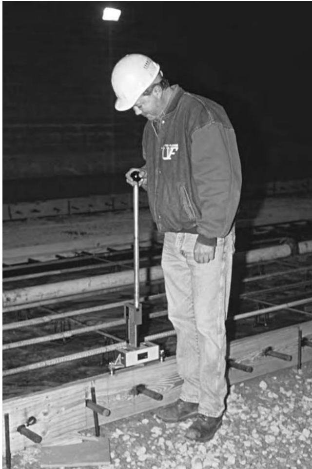
Figure 11.11 Using an electronic level to check a timber form on a superflat job
