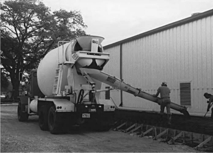
Figure 11.1 Discharging concrete straight from the ready-mix truck into the forms
