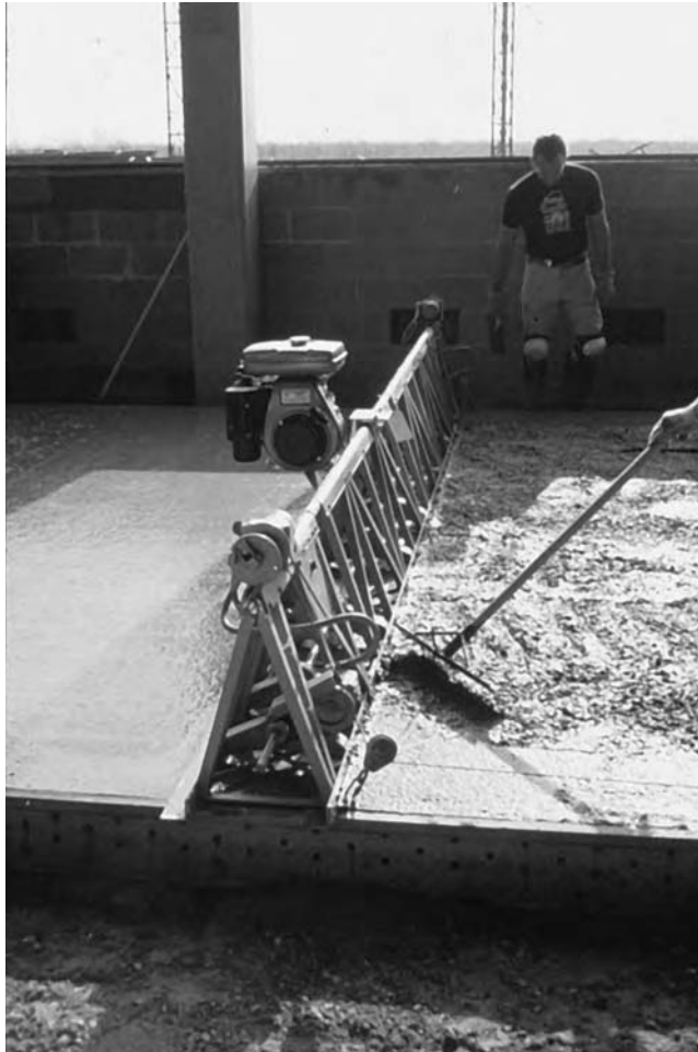
Figure 17.4 Truss-type vibrating screed
