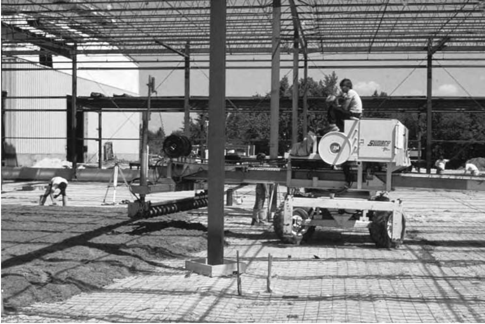
Figure 11.10 Laser screed
