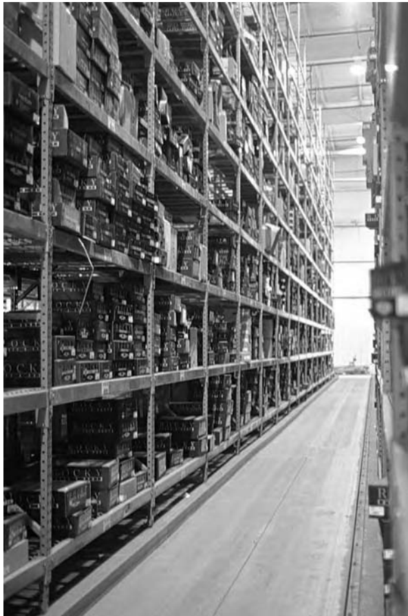
Figure 3.3 Heavy-duty shelving in a very-narrow-aisle (VNA) warehouse
