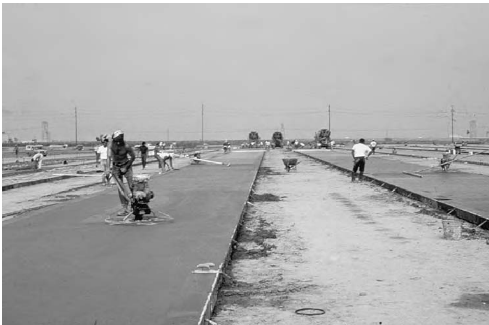
Figure 11.5 Narrow-strip construction is standard for superflat floors
