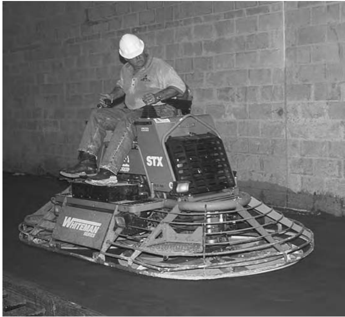
Figure 17.8 Riding trowel machine fitted with float pans
