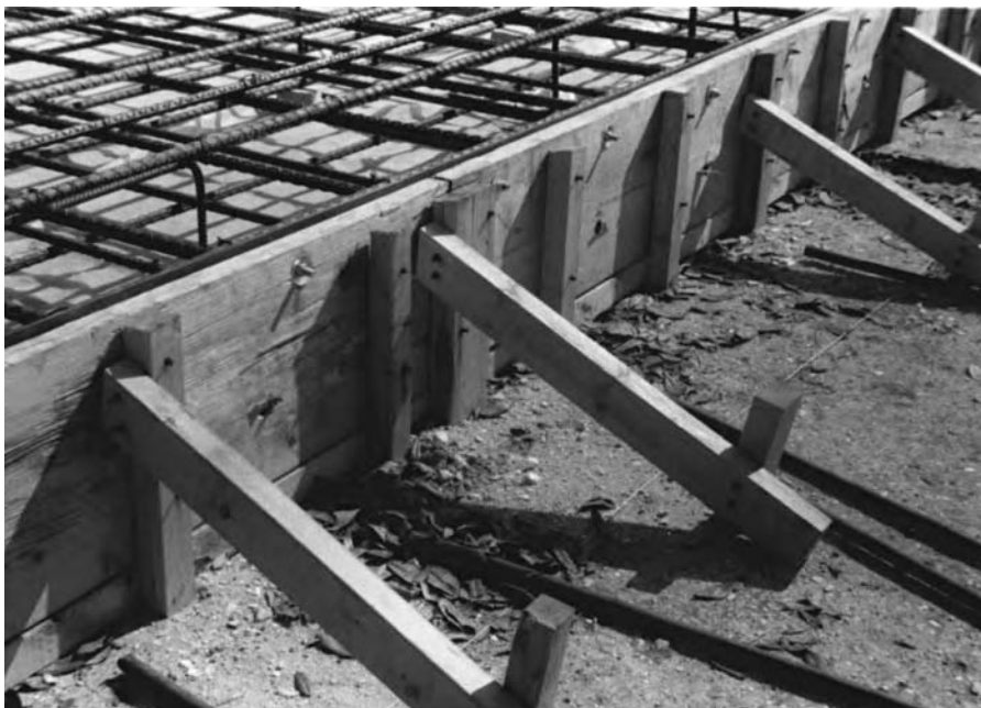
Figure 11.13 Heavily braced timber form
