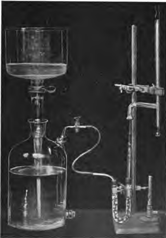
Fig. 27. Formation of water on burning hydrogen.
